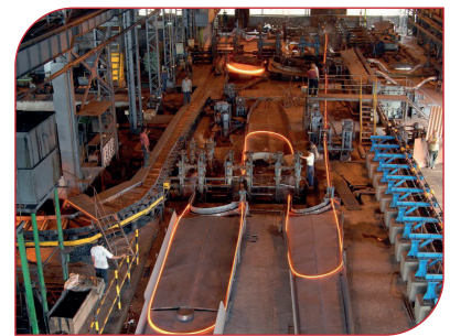
Jairaj Steel Plant Andhra Pradesh
