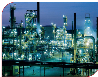
Reliance Refinery Jamnagar, Gujarat
